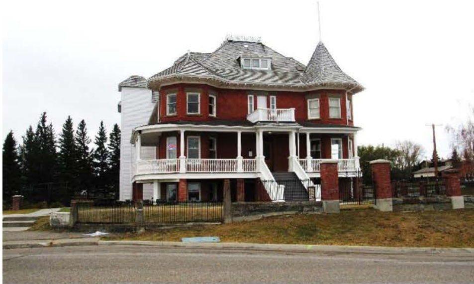
General view of the Site building.
