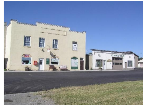
Figure 4. Cowley's main street. Source: Village of Cowley
