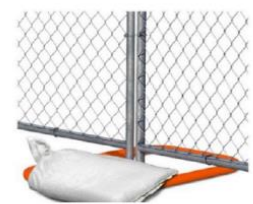
Temporary Fencing on Moveable Bases
